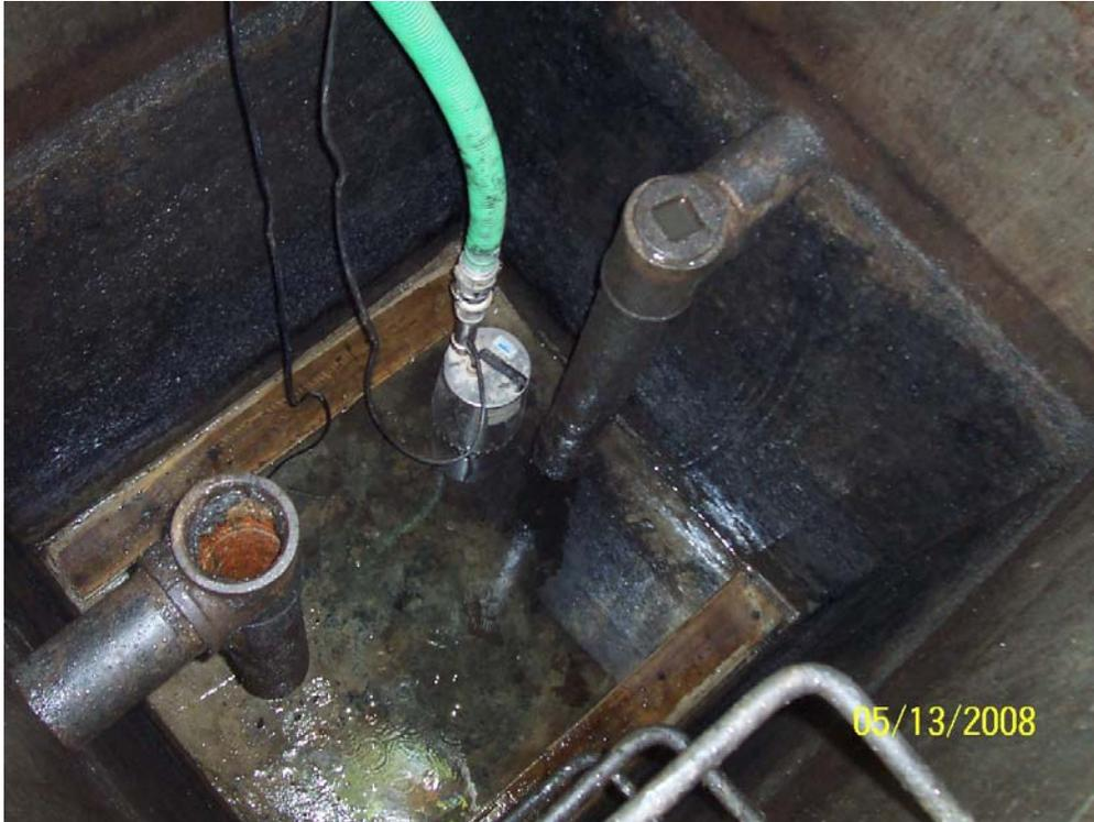
Photo 3 - Sump pump installed in Building 45 vault to remove liquids after cleaning.
