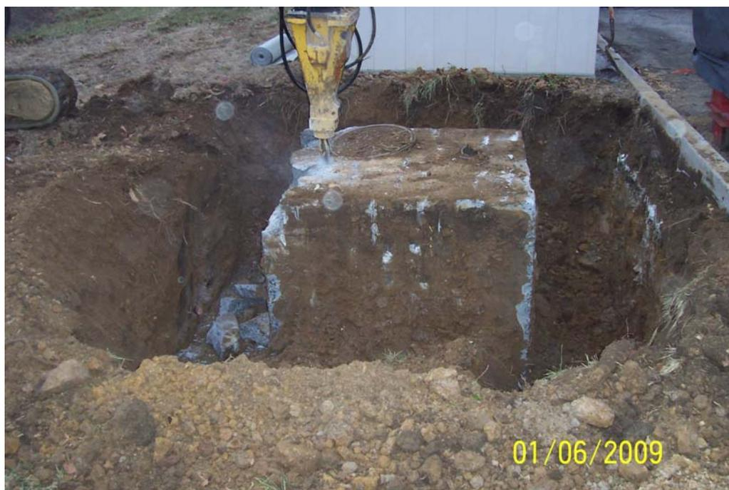
Photo 8 - Excavating Building 45 Vault and breaking concrete with jack hammer.
