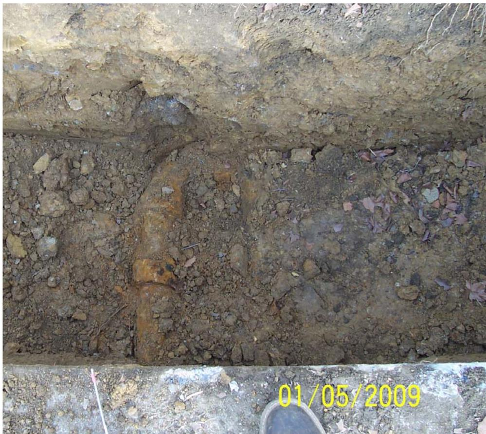
Photo 7 - Influent pipe from Building 45 into vault.
