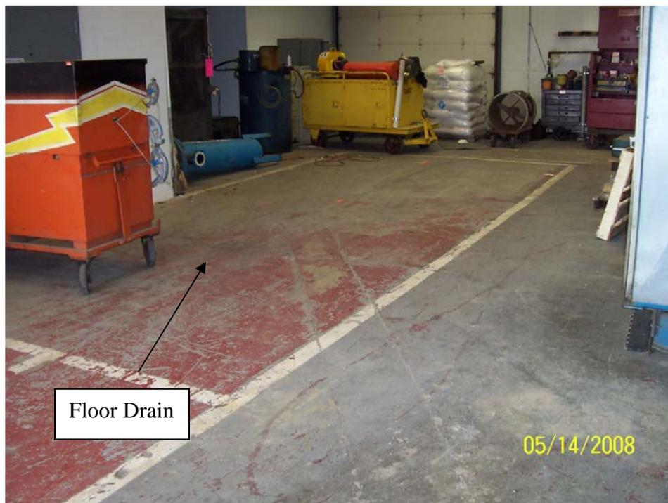
Photo 6 - One of the 3 floor drains in Building 45 that were cemented shut as part of the vault closure procedure.
