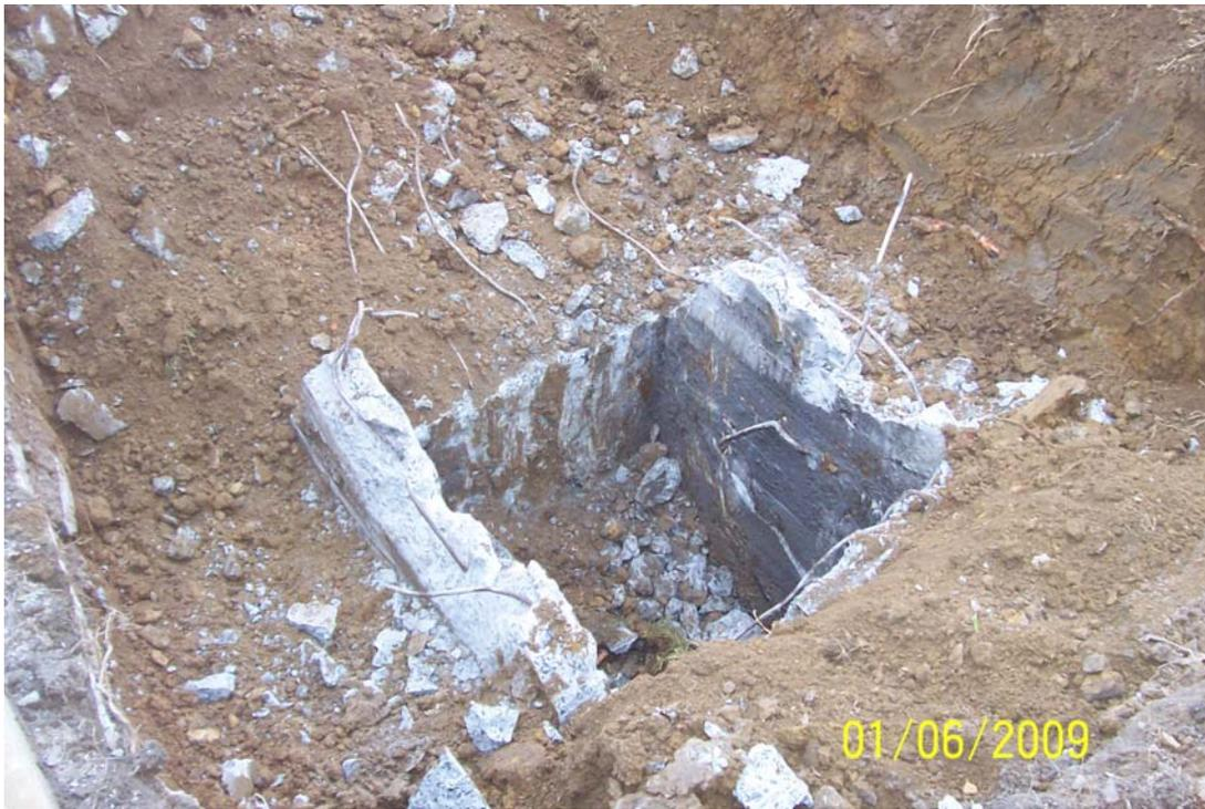
Photo 9 - Vault with top removed.
