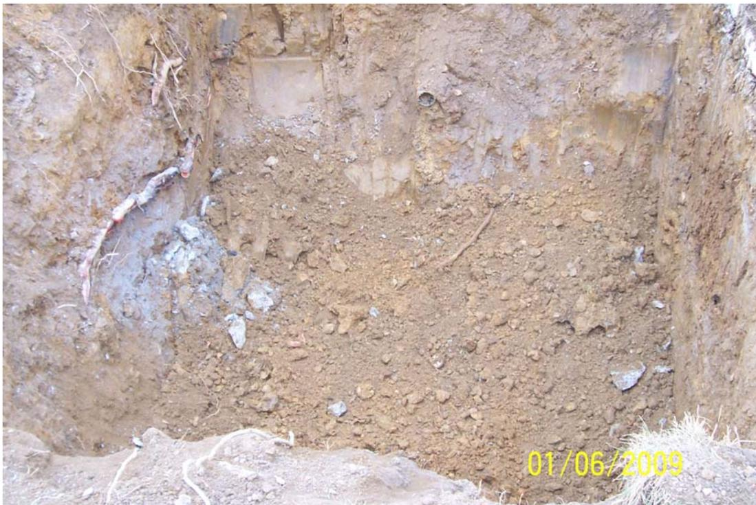
Photo 10 - Vault removed from excavation. Influent pipe visible on north side of excavation.
