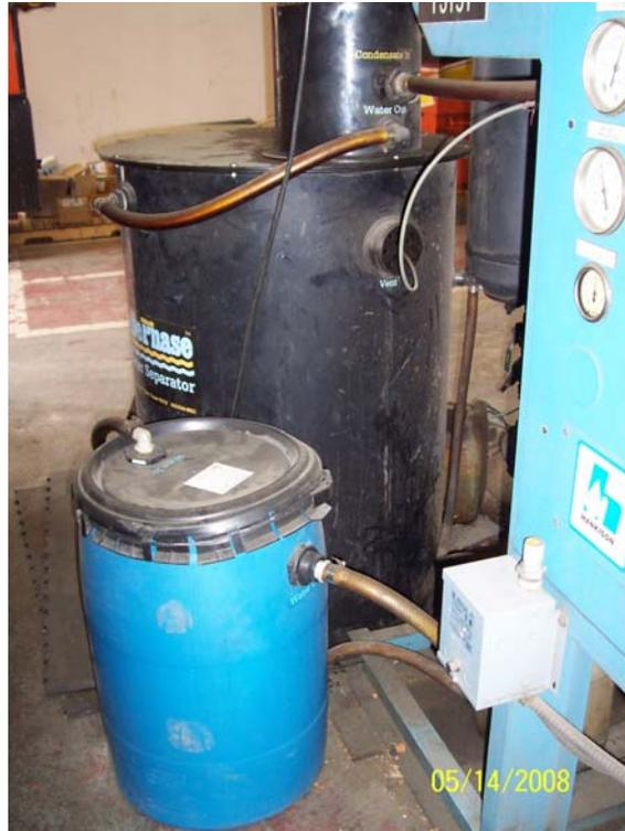
Photo 5 - Condensate knockout tank that was the source of water draining into the vault following cleaning. This water was redirected with a hose to discharge into floor drain in men's bathroom during the closure of the vault.
